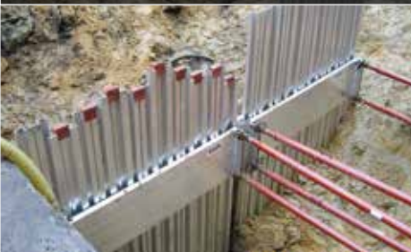
LITEBOX manhole shoring system
