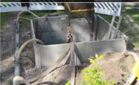
LITEBOX manhole shoring system
